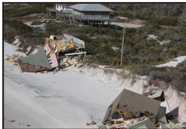
Damage was widespread on St. George Island after Hurricane Dennis in 2005. (Aerial photo by Tom Meares)
